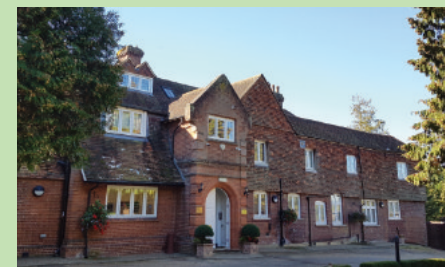
Above and top: RES HQ – The Mansion House, St Albans.
