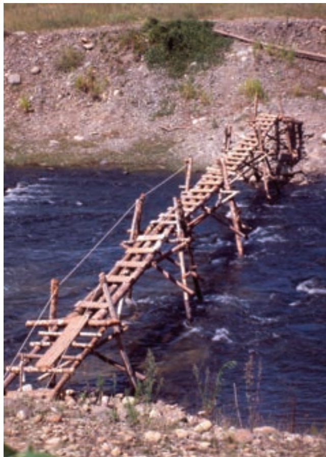
Fig. 4. The deluxe Phase 2 bridge (photo: John Tennent).
